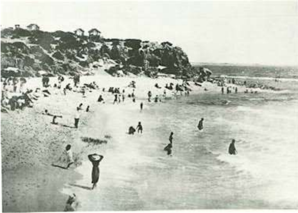
Figure 14: Mudurup Rocks with structures on headland (circa. 1900). 'Cottesloe Beach was already a popular destination in the early 1900's. The completion of the jetty in 1908 added to its popularity.' The addition of the Cottesloe groyne in 1960 further increased the popularity of this icon beach of Western Australia. (Photo courtesy, Town of Cottesloe CPM00961)
